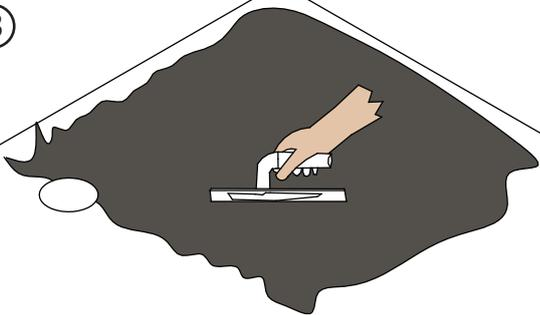
Install the shower tray on a 15mm depth of weak cement mix (sand/cement ratio 5:1). Tile adhesive can be used as an alternate to sand or cement. Please note if using water based adhesives, to enhance the bonding it is suggested that a suitable primer is applied to the base of the shower tray before installation.
